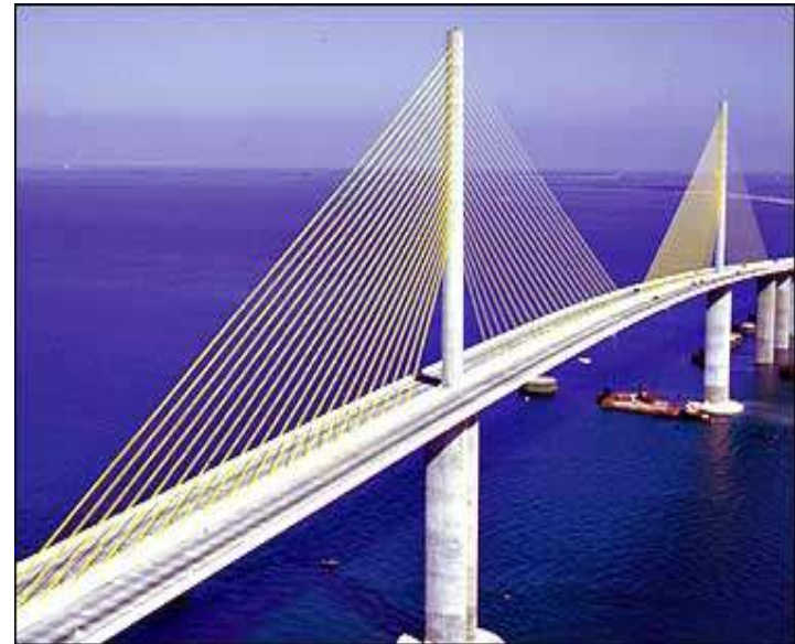
Foto: Sunshineskyway Bridge, Florida
